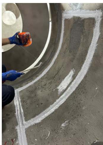
Rebuilding weld seams with Belzona 1511
