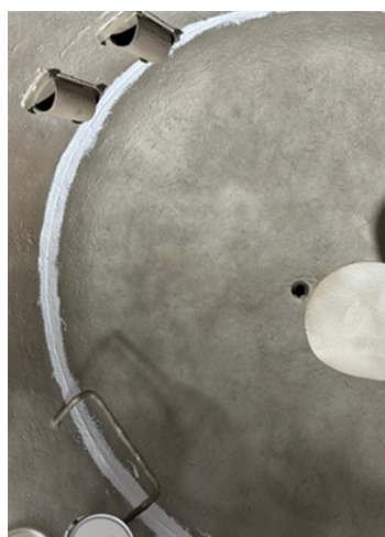
Rebuilding vessel weld seams with Belzona 1511
