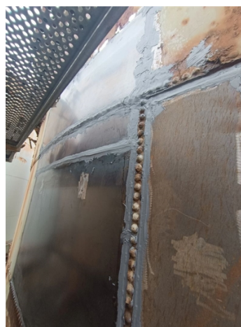
Belzona 1161 applied to thinner wall damaged areas
