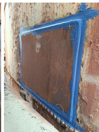
Belzona 7311 used to bond thicker plates
