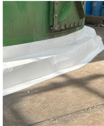
After applying Belzona 3111 Flexible Membrane
