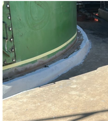
Rebuilding the concrete with Belzona 4111 Magma-Quartz
