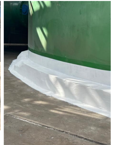
After applying Belzona 3111 Flexible Membrane to vessel base
