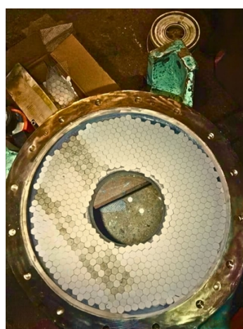
Installation of Belzona 9811 Alumina Tiles completed
