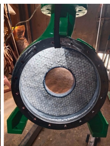
Completed installation and grouting of Belzona 9811 Alumina Tiles
