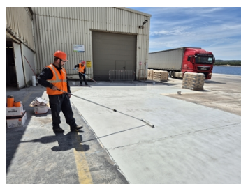
Application of Belzona 5231 and Belzona 9221 in progress
