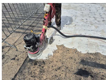
Surface preparation in progress
