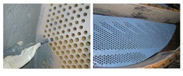
The protection of the inner surface of the pipes was done by gluing steel inserts inside the pipes. Top layer of Belzona 1341 product.
