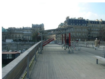
Non-disruptive application in 2000
