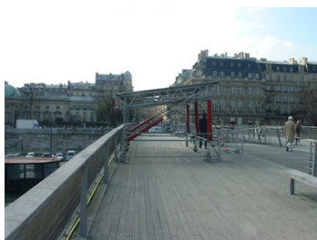
Non-disruptive application in 2000
