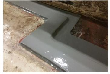
Repair overcoated with Belzona 5831 for corrosion protection
