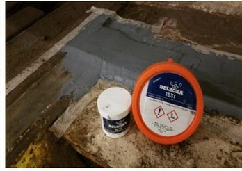
Belzona 1161 used to rebuild the damaged area
