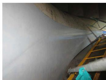
Belzona 1311 Ceramic R-Metal topped with Belzona 1341
