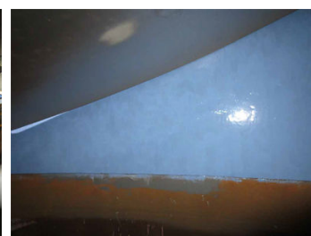
Second and final coat of Belzona 1341
