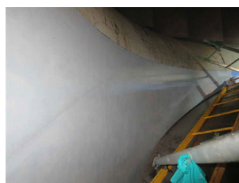
Belzona 1311 Ceramic R-Metal topped with Belzona 1341
