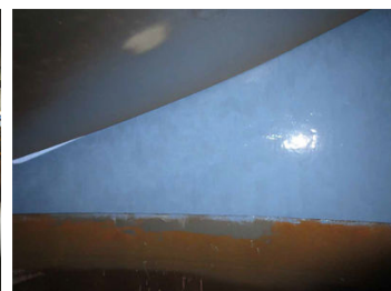
Second and final coat of Belzona 1341
