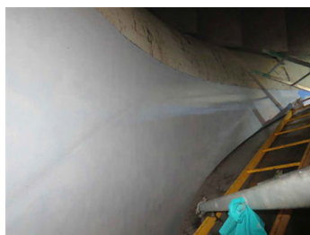
Belzona 1311 Ceramic R-Metal topped with Belzona 1341
