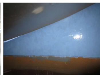
Second and final coat of Belzona 1341
