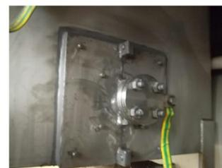
Plates and Belzona Applied to Affected Area; Reading for 2 Hour Curing
