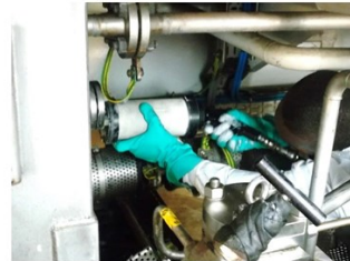
Injecting Belzona Compound to fill Any Gaps Between Plates and Tank
