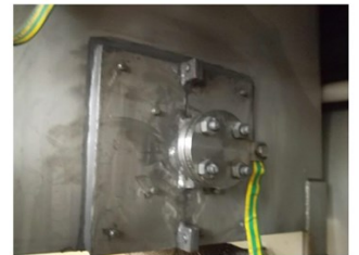
Plates and Belzona Applied to Affected Area; Reading for 2 Hour Curing
