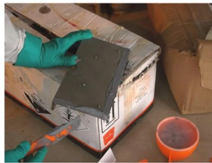
Applying Belzona Compound to Metal Plates
