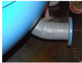
Plate bond &amp; wrap applied
