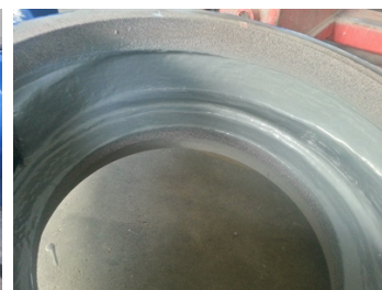
Repair detail with Belzona 1812 and 1391 products
