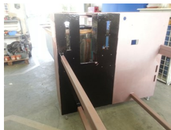
Coating selected impacted areas by Belzona 5811
