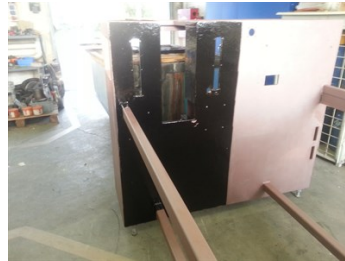
Coating selected impacted areas by Belzona 5811
