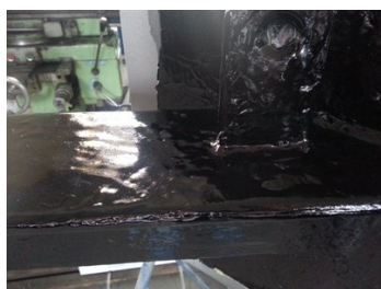
Belzona 2111 application
