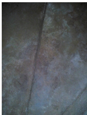
Corrosion on the welding seams
