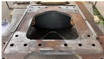
Power tool preparation on the damaged surfaces
