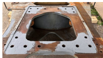
Belzona 1111 built up proud of casing
