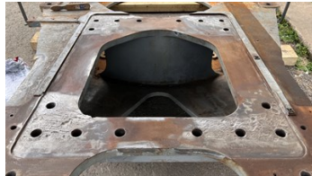
Power tool preparation on the damaged surfaces
