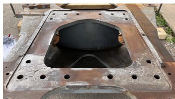
Power tool preparation on the damaged surfaces
