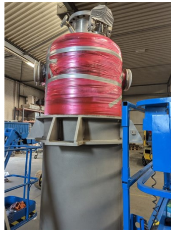
Application of Belzona SuperWrap II
