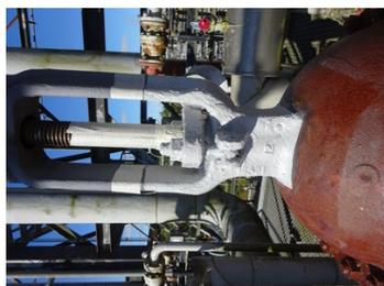
1st coat of Belzona 3412 applied
