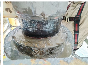
Hole repaired with SuperWrap II.
