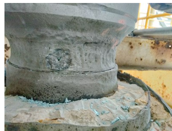
Surface after grit blasting.
