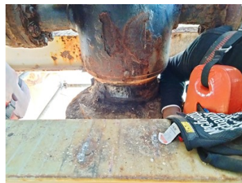
Defect located and prepared for plug with Belzona 9611.
