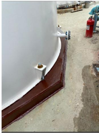
Belzona 4311 applied to provide excellent chemical resistance to the tank base.
