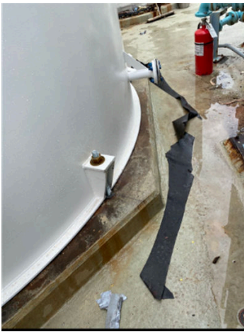
Previous coating was removed.
