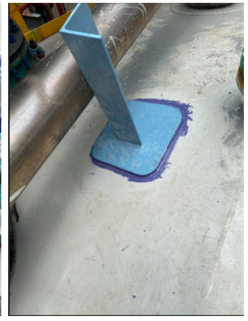
Belzona 7311 to bond pipe supports to the top of the tank.
