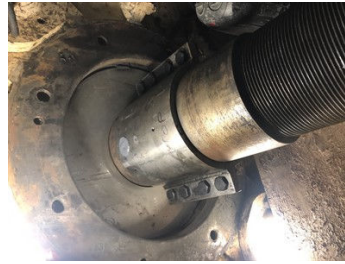
Mold in place and injection of Belzona 1321 Ceramic S Metal complete
