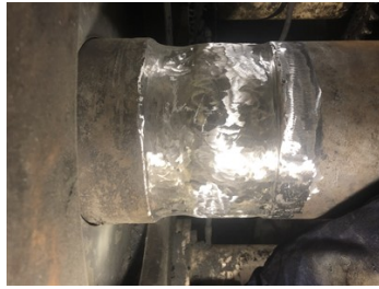
Surface prep in progress
