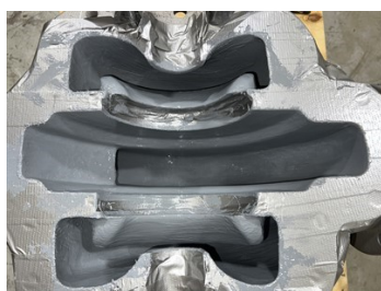
First coat of Belzona 1321 (grey).
