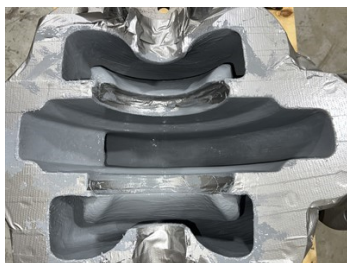
First coat of Belzona 1321 (grey).
