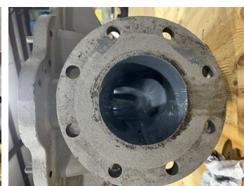
Second view of Belzona 1321's second coat.
