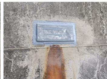
Plate bonded in place with Belzona 1161
