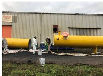
Pipework mid-application of Belzona 5811.
