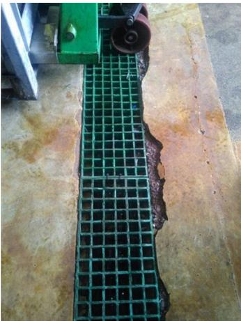
Loose grates and crack shoulders, requiring rebuilding using 4181
