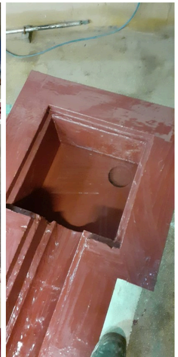
Completed 4181 concrete repairs and 4331 coating
