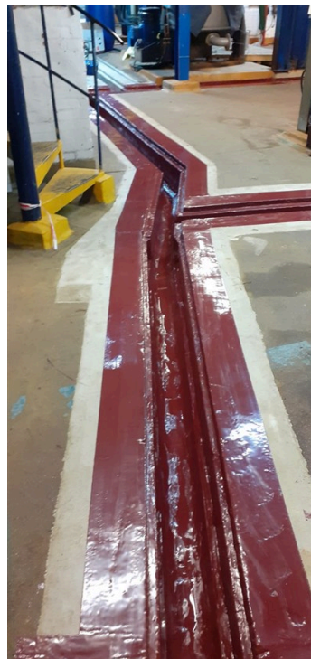
Completed 4181 concrete repairs and 4331 coating
