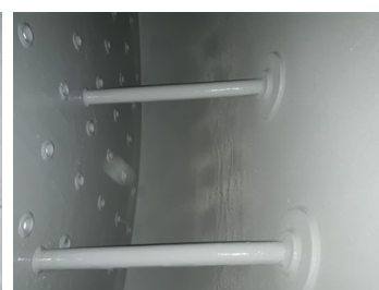
Application completed and protected tank inner surfaces
