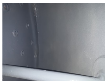
Initial coat of Belzona 1321 being applied
