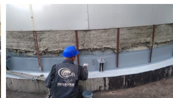
Application du Belzona 5811 to protect the plate bond against the environment.
