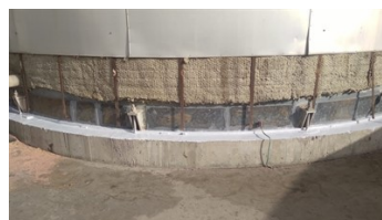
Plate bond reinforcement on the lower part of the tank.
