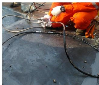
Inject Belzona 5811 to cold bond the doubler plate located
