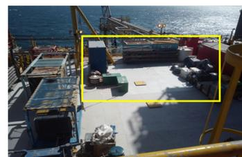
Once the bonding application of the doubler plates is completed, the deck top was coated with Belzona 5231 and 5233
