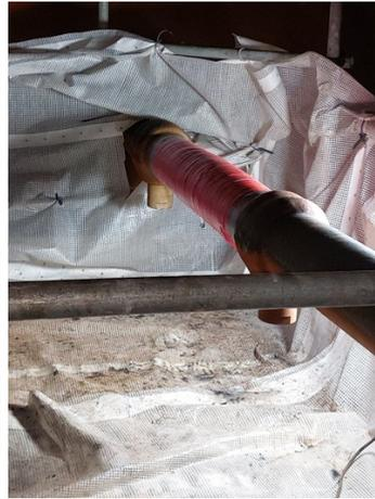
Damaged area reinforced using Belzona Super Wrap 2
