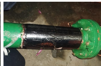
Strengthen pipe section
