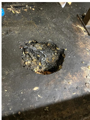
Deep corrosion in areas of spillage
