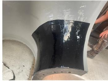
Post substrate rebuilding, the first coat of Belzona 1341 and Belzona 2141.
