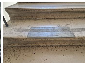
Loss of thickness on a stair due to 120 years of wear, represents a risk of falling and injury.
