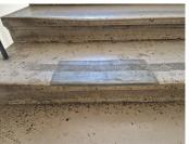
Loss of thickness on a stair due A stair rebuilt to its original to 120 years of wear, represents a risk of falling and injury.
