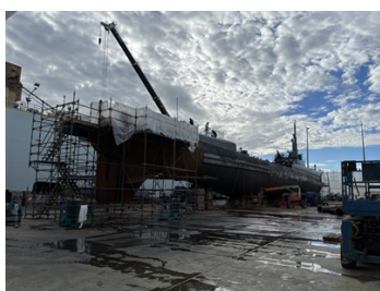
USS Bowfin on dry dock being refurbished.
