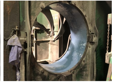
Coating of Belzona 1321
