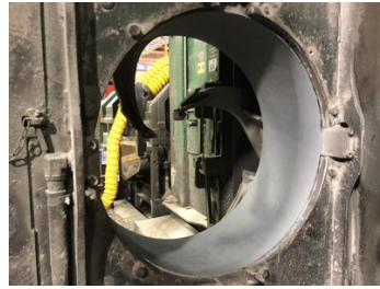
Resurfacing with Belzona 1311
