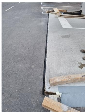
Expansion joint cleaned and conditioned with Belzona 4911
