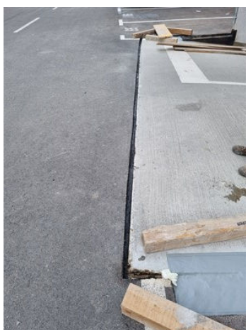
Expansion joint cleaned and conditioned with Belzona 4911
