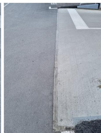
Situation after 7 months, with Belzona sealants still intact and in perfect condition.
