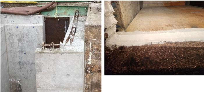
Steel plate, uncut, before the concrete floor and surrounding building were installed. Sealed seam, concrete-steel-concrete.
