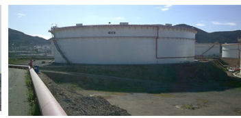
One of the tanks with the tank base sealing system installed.
