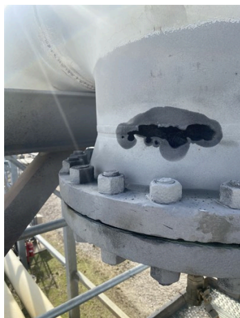
Clamp removed and vapor blaster used.
