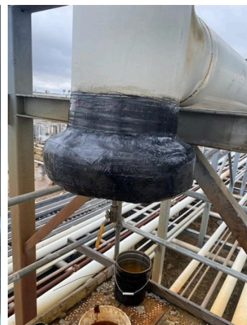
Finalized SuperWrap II application.
