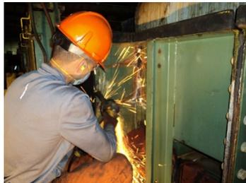
Surface preparation with a grinder to bare metal
