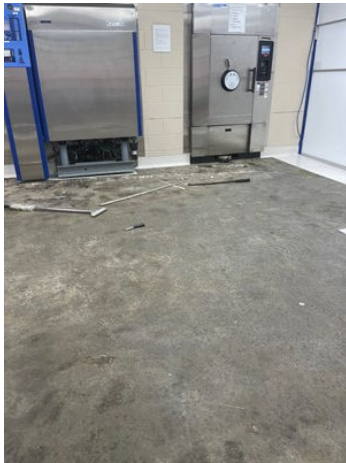
Vinyl Flooring Removed
