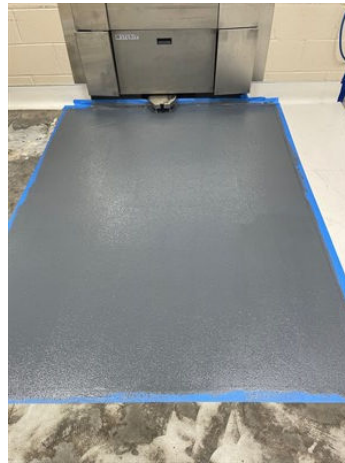
Belzona 1321 applied in front of Cartwash units
