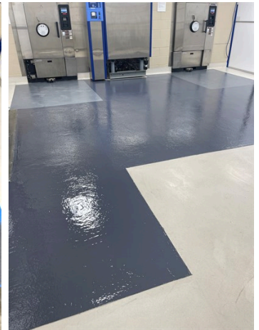
Belzona 4311 applied to rest of the area
