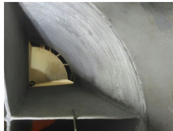
Belzona 1111 used to repair and rebuild the valve's body.
