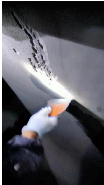
Pitting corrosion before repair
