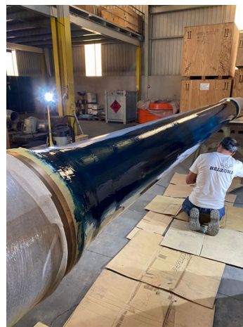
3.) 1st coat of Belzona 2141 being applied
