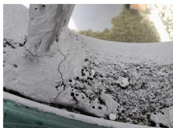
Before application: internal pitting damage
