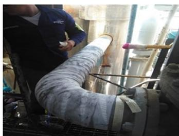
First layer of Belzona 1161 and reinforcement mesh.
