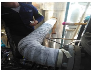
First layer of Belzona 1161 and reinforcement mesh.
