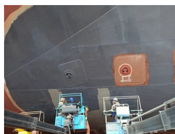
The first coat of Belzona 4311 (grey) was being applied
