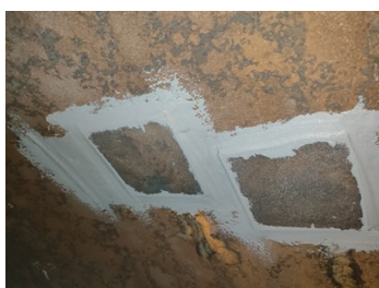
Use Belzona 1111 to repair pipe leakage
