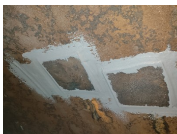
Use Belzona 1111 to repair pipe leakage
