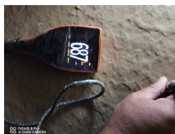
DFT test after applying two coats of Belzona 5811
