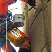
Rope access and a lightweight Completing the works repair polymer was the most preferential choice due to access difficulties
