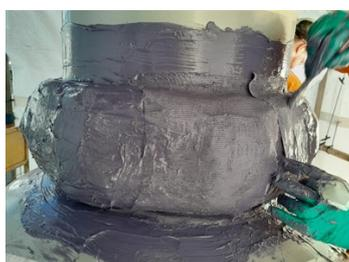
Wetting out of the Breather Membrane and vertical application of Reinforcement Sheets (Belzona 9341) using Belzona 7311.
