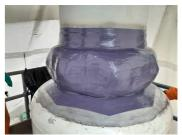
Post-application of 5x wraps of Final application after a further encapsulating layer of Belzona 7311.
