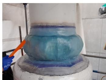
Post-application of 5x wraps of reinforcement sheet (Belzona 9371) and Belzona 1981 resin.
