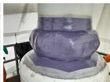
Final application after a further encapsulating layer of Belzona 7311.
