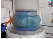
reinforcement sheet (Belzona 9371) and Belzona 1981 resin.
